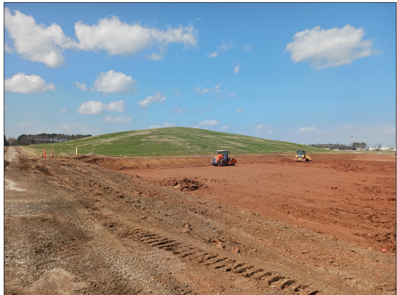
Photo No. 5 Looking west at the northern slopes of Areas 1-3.
